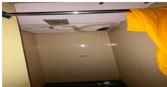
Mould on ceiling tile (washroom 3042A)
